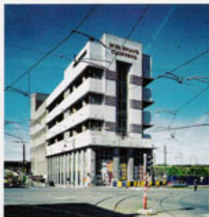
Site of the future Wiels Contemporary Art Center in Brussels.
